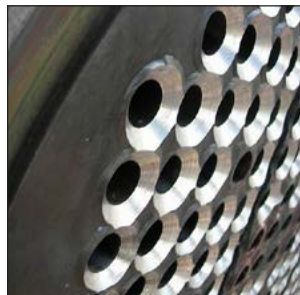
Completed strength weld removal.
