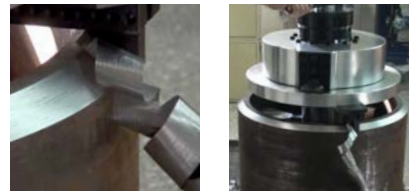
Machining pipe 24" schedule 160
