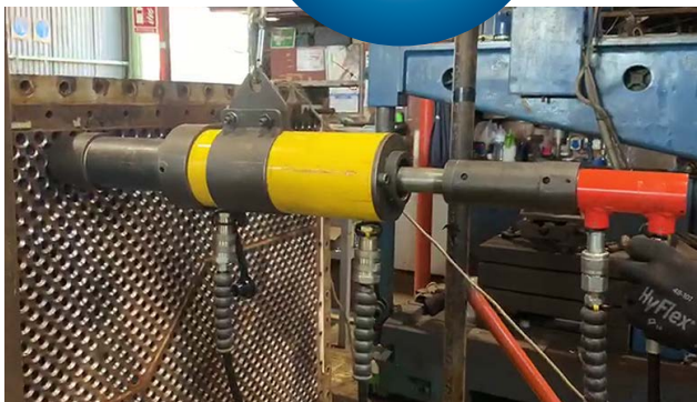
Puller in the application of 1" GA 14 tube in 4" tube sheet.
