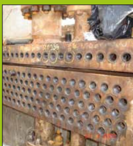
FinFan cooler before a maintenance
