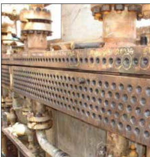
FinFan cooler before a maintenance
